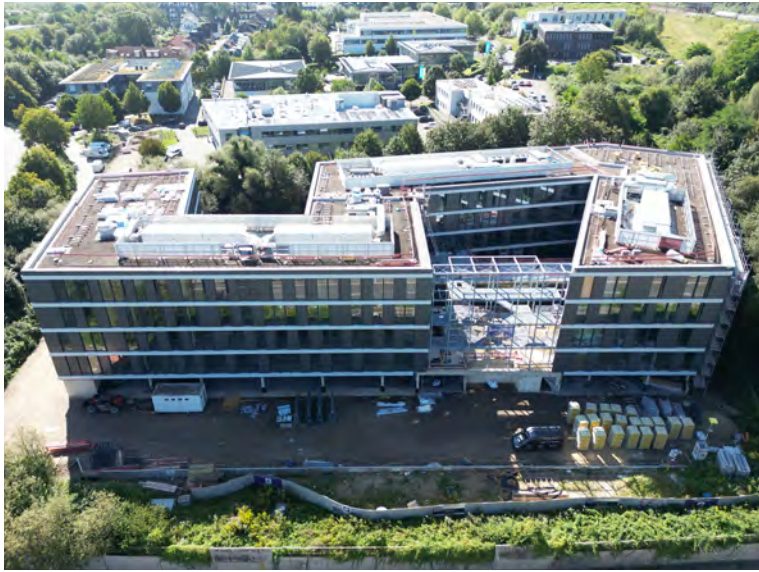
■ Das Office West in Aachen
